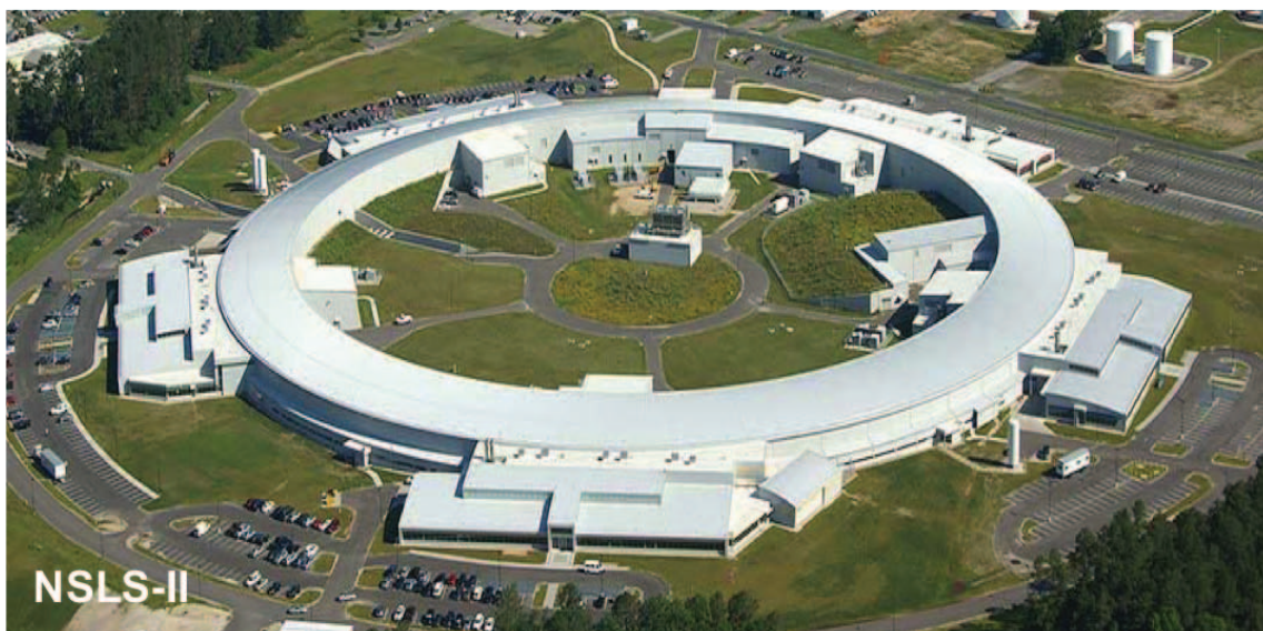
Figure 1: NSLS-I (top) and NSLS-II (bottom) facilities at Brookhaven National Laboratory. The NSLS-II is 5 times the size and 10,000 times brighter than the NSLS.
