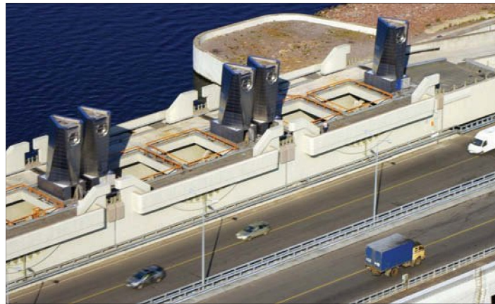
Sluices: Pistons in stainless steel housings push the sluice gates down
