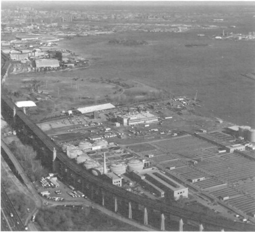
Dewatering facility on Wards Island. East River to the east, New York Central Railroad to west, Bronx in background. Photo by Bernstein Associates, Mount Vernon, NY.
